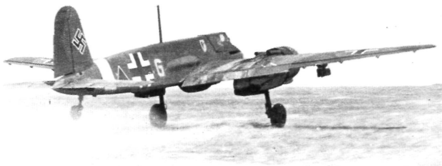
The near-triangular fuselage section of the Henschel Hs 129B, adopted to minimise frontal area to improve survivability, is clearly seen from this angle. It was the first of the 'big gun' anti-tank aircraft, but its flying qualities were poor and its engines unreliable. (Bruce Robertson)
